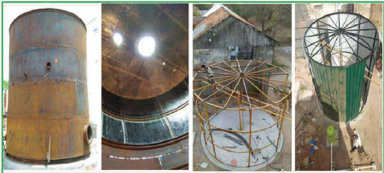
Mild Steel (MS + FRP) - 1000 KG Biodigester Plant
